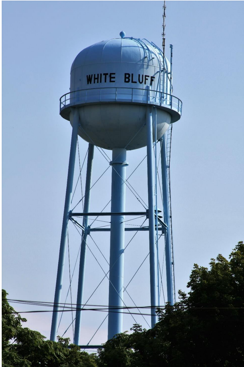
Figure 9: White Bluff Water Tower, Downtown, White Bluff, TN.
