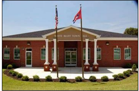
Figure 20: White Bluff Town Hall, Hwy 70, White Bluff, TN.
