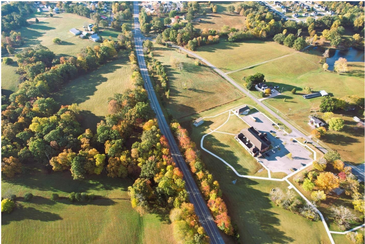
Figure 31: Drone view of Hwy 47N looking south, White Bluff, TN
